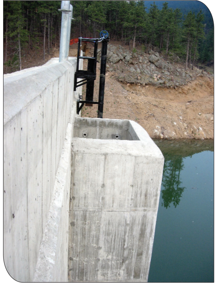
Service spillway uncontrolled drop inlet
